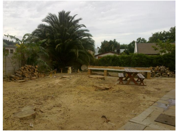
The cleared area ready for renovation
