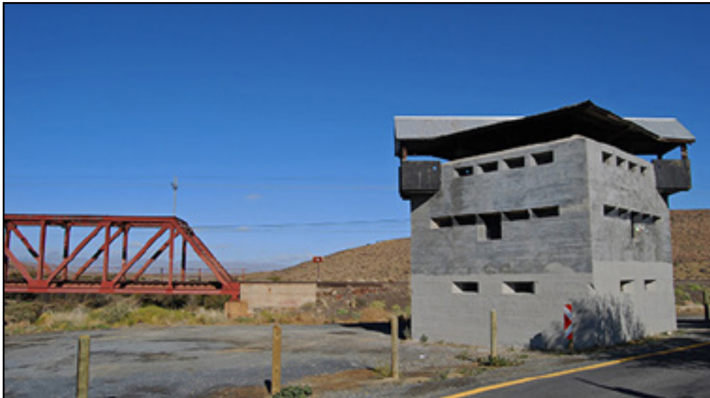
BLOCKHOUSE: One of the nearly 8,000 blockhouses that were built during the Second Anglo-Boer War. This one is near Lainsburg.
