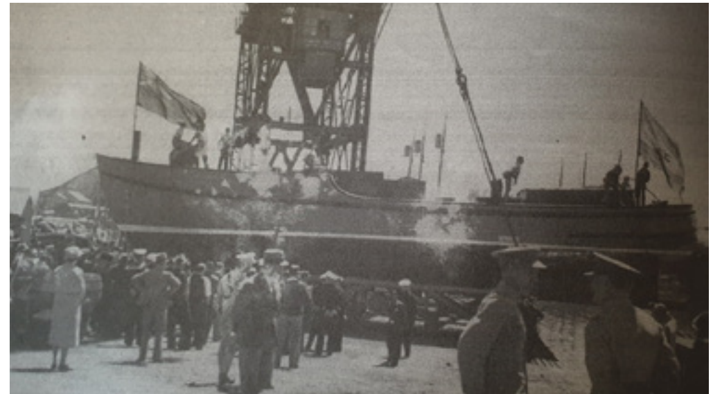
LAUNCHED: The Isie is launched from the Cape Town builder’s yard of Louw and Halvorsen on 12 May 1941.
